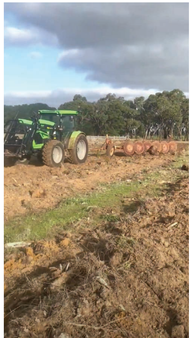
Pederick Rake used to windrow stumps.
